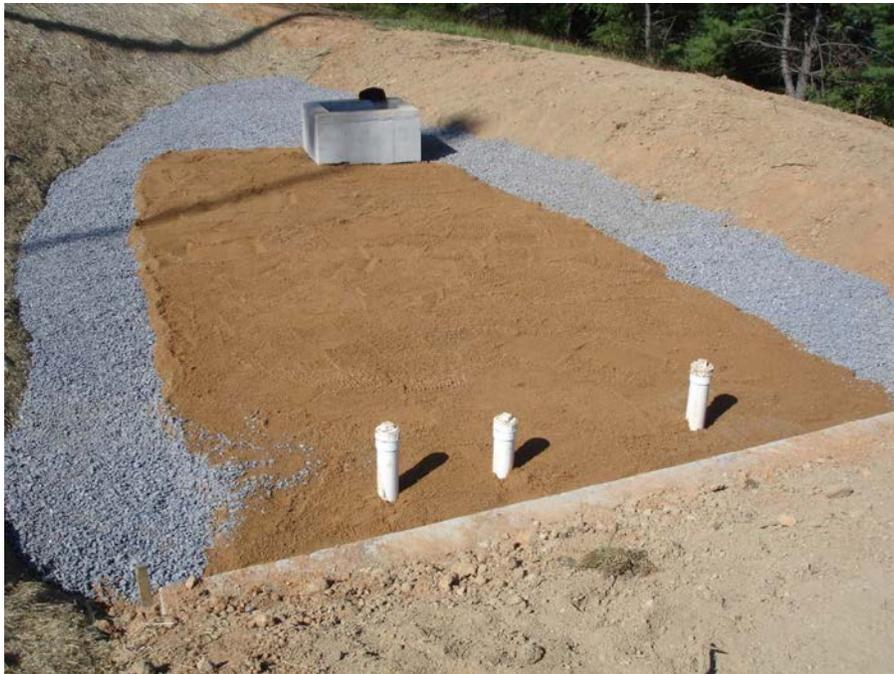
Figure 8. Shows a sand filter that is located below the turf fields at UREC. There are three underlying drains for the water once it flows through the sand bed.
