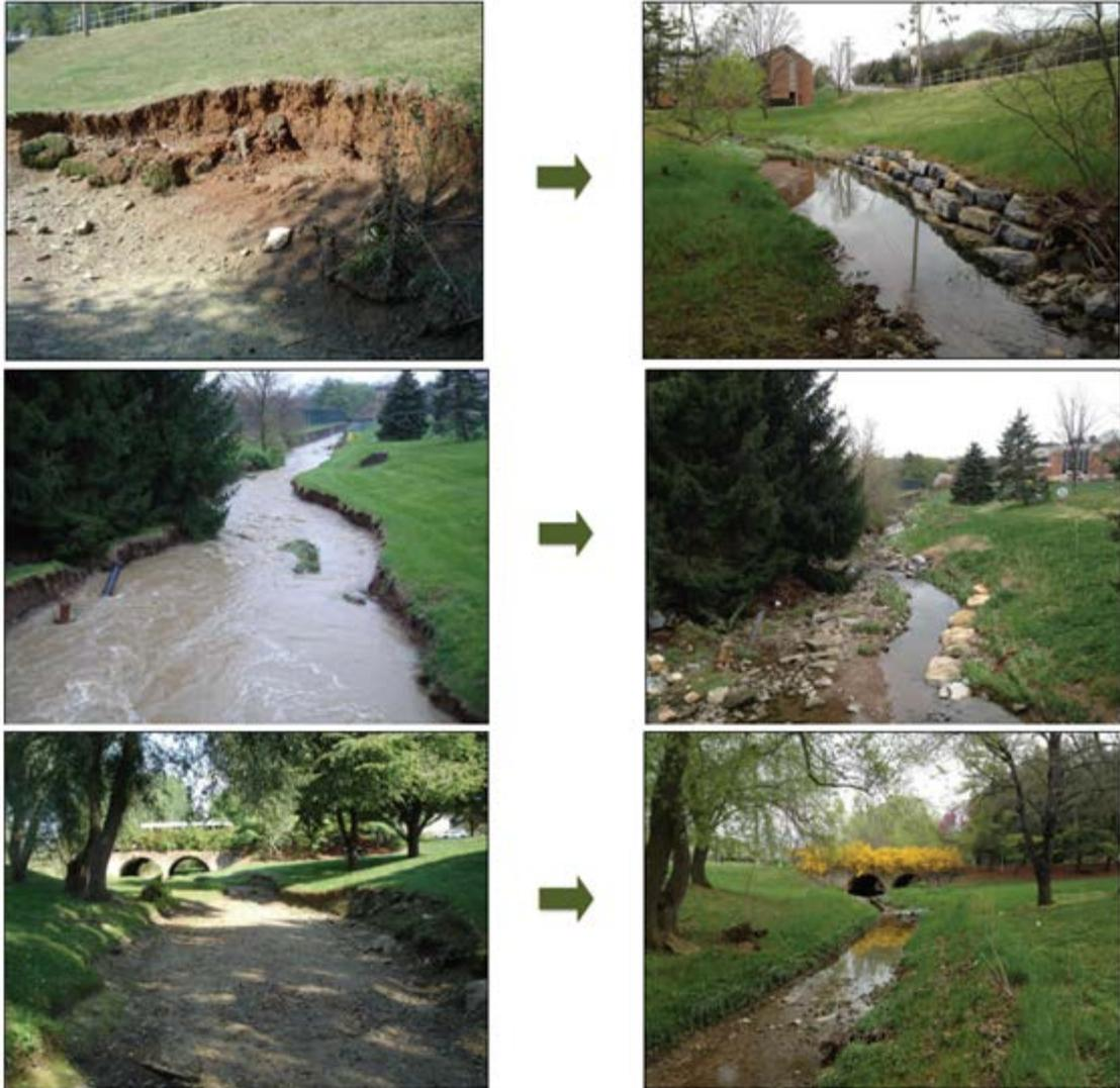
Figure 2. Shows Siebert Creek before and after the restoration. The pictures are beside the C4 lot (top), by the Hillside Bridge (middle), and by the Paul Street Bridge (bottom). These techniques can effectively minimize the effects of storm water on the creek bed and banks. Photo courtesy of HR Horizons.
