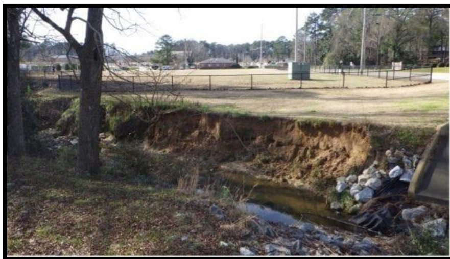
Figure 9. Typical erosion observed on urban stream banks. (Alabama Cooperative Extension) (7)
