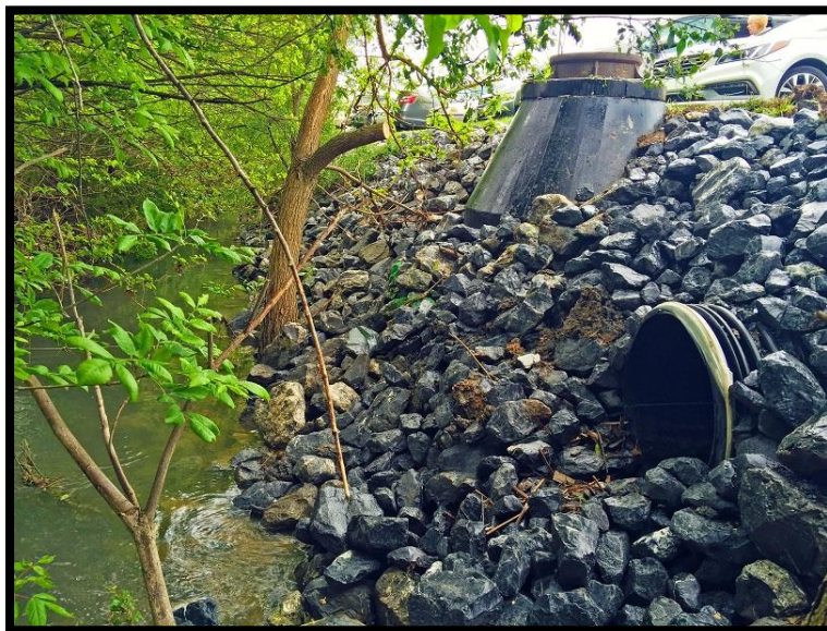
Figure 11. Sewer manhole next to stormwater outfall on hardened stream bank on campus. (Photo: Dale Chestnut)
