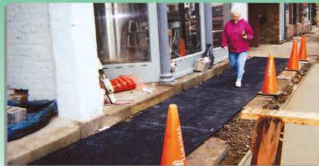
VersaMATS lock together to form continuous walkway
