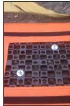
Install base with 2 to 4 anchors as needed.
