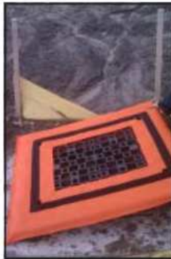
Install Grate Pyramid base over grate.
