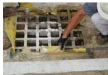
To remove Siltsack®, clean area around grate and slide rebar through Siltsack® pockets.
