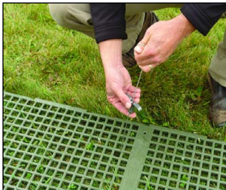
Figure 6. Install Anchor Brace/Gripple
