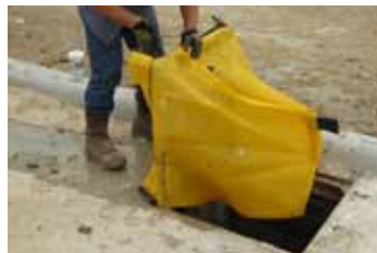
Slide Siltsack® over opposite side of grate.
