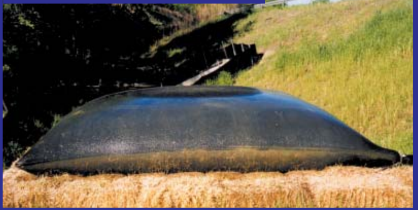
Hillside Installation on Straw Underlayment
