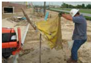
To clean Siltsack® attach rebar through empty loops at bottom and lift to empty.
