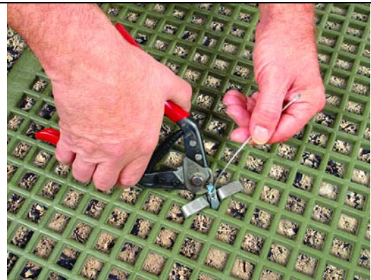
Figure 10. Cut the cable flush with the Gripple
