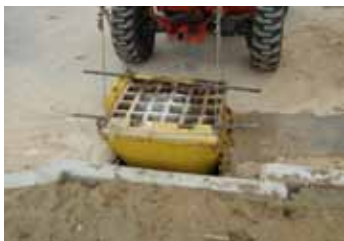
Slowly remove Siltsack® from inlet.
