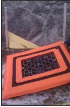
Install Grate Pyramid base over grate.
