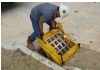
Replace Siltsack® and grate inlet into recess.
