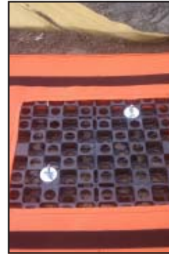
Install base with 2 to 4 anchors as needed.
