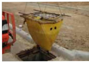
Removed Siltsack® is now ready for cleanout.
