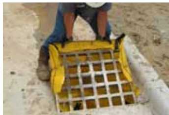
Slide Siltsack® over one side of grate.
