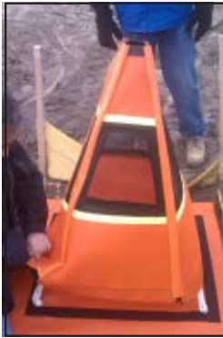
Slide tower filter over frame.
