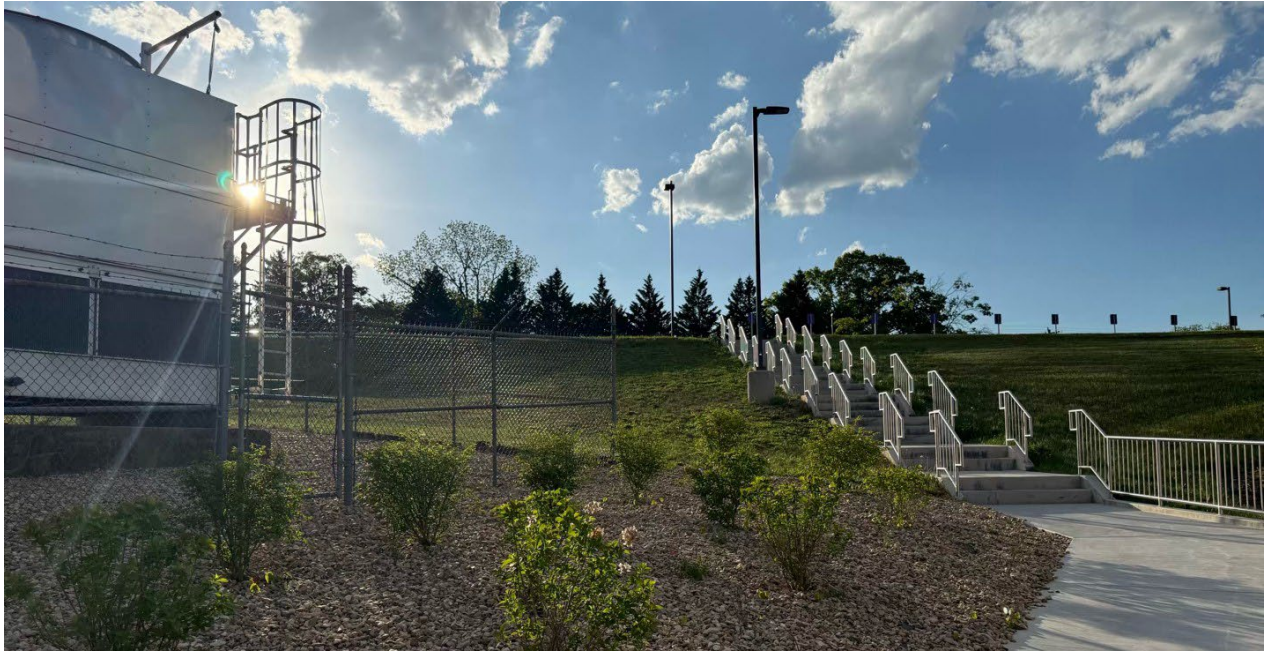
Figure 12: View facing north toward South Willow Street
