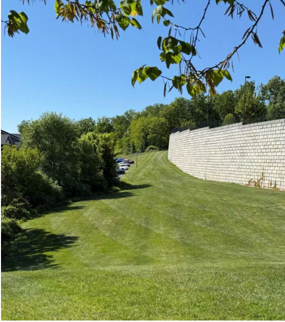
Figure 13(a): View facing northwest from Devon Lane
