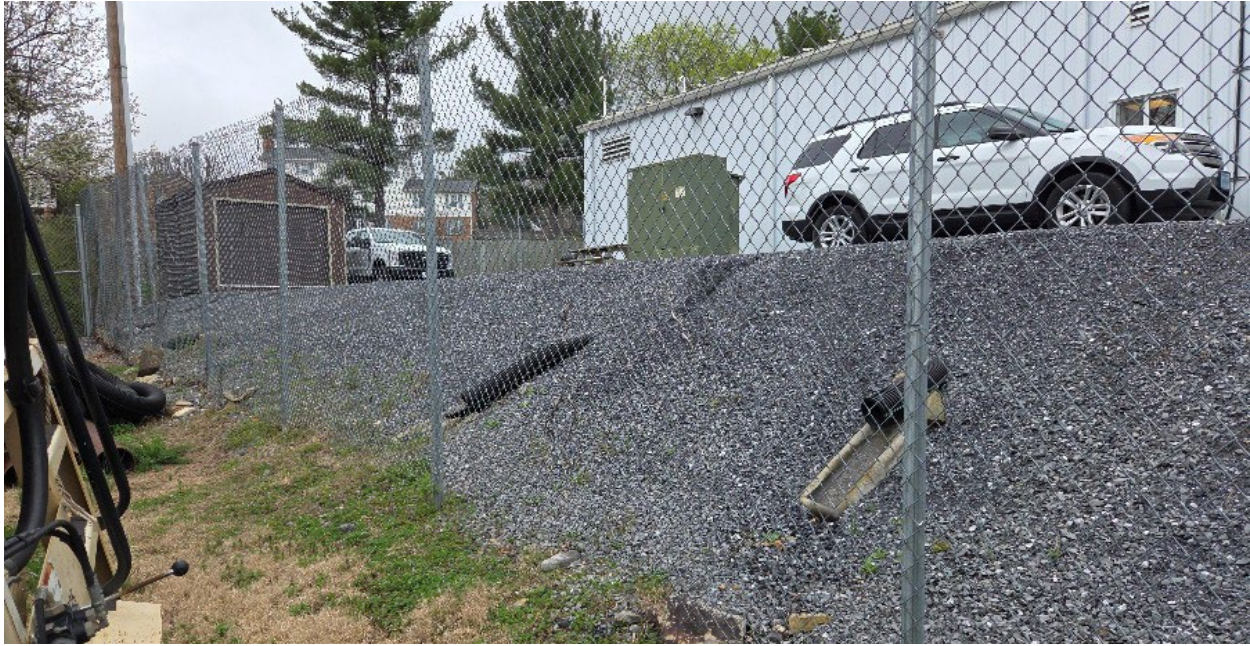
Figure 34: View facing north toward the Alternate Fuel Building
