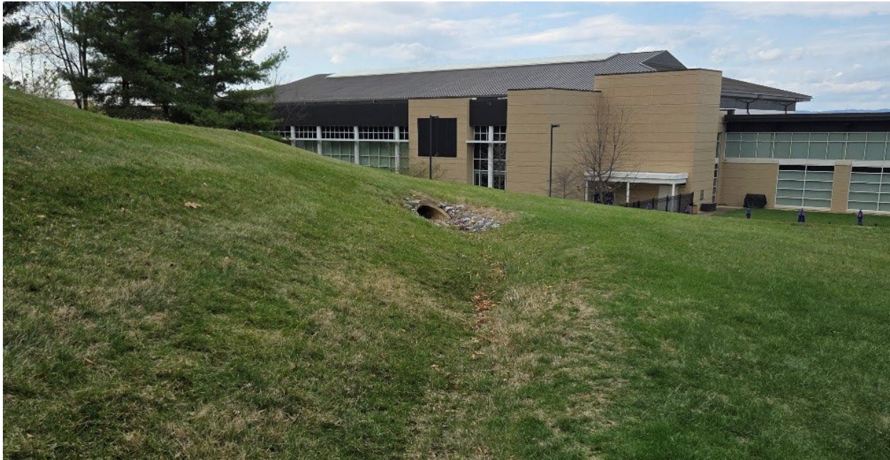
Figure 25: View facing north toward UREC, showing the existing grass channel outlet
