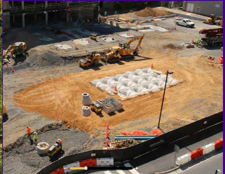
Underground detention facility installation.
