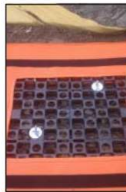
Install base with 2 to 4 anchors as needed.
