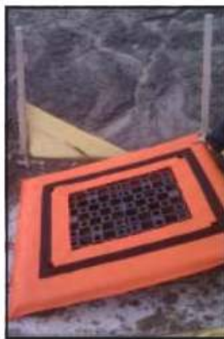
Install Grate Pyramid base over grate.
