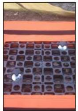
Install safety caps on anchors.
