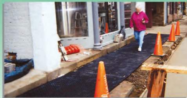
VersaMATS lock together to form continuous walkway
