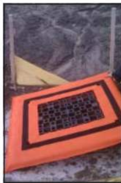
Install Grate Pyramid base over grate.
