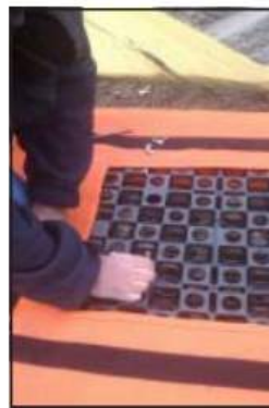
Install anchors.
