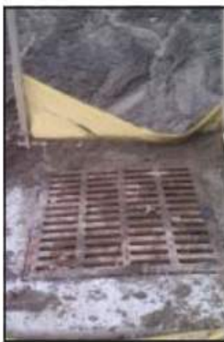
Standard drop inlet grate.
