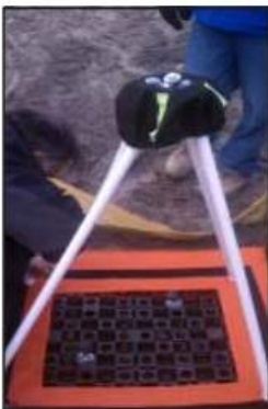
Install tower frame.
