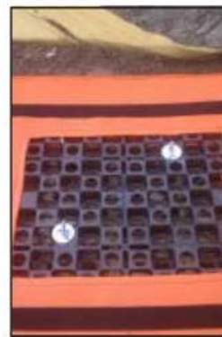
Install base with 2 to 4 anchors as needed.
