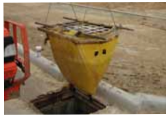
Removed Siltsack® is now ready for cleanout.
