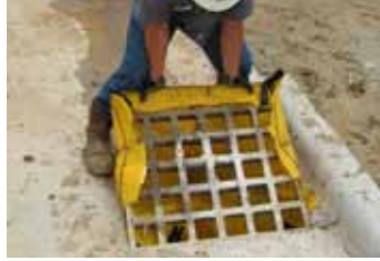
Slide Siltsack® over one side of grate.
