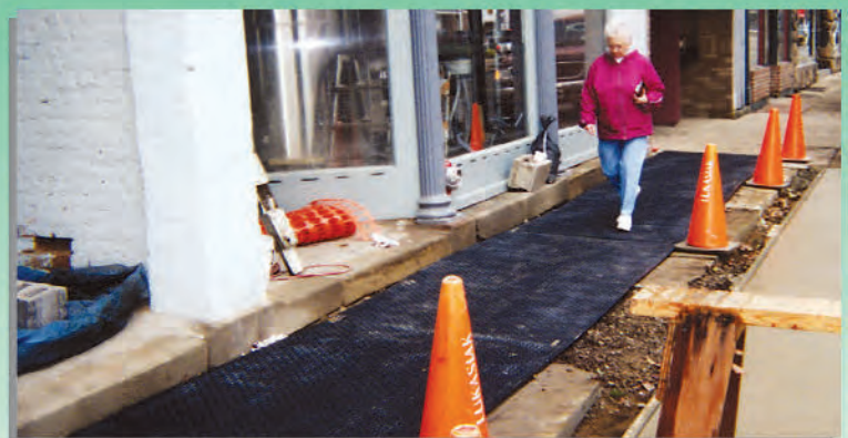
VersaMATS lock together to form continuous walkway
