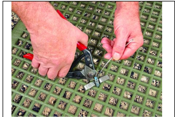
Figure 10. Cut the cable flush with the Gripple
