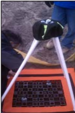
Install tower frame.
