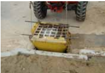
Slowly remove Siltsack® from inlet.
