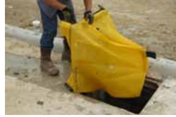
Slide Siltsack® over opposite side of grate.
