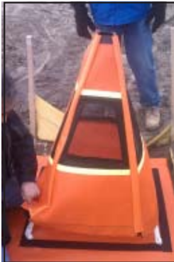
Slide tower filter over frame.
