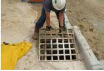
Remove grate from catch basin.
