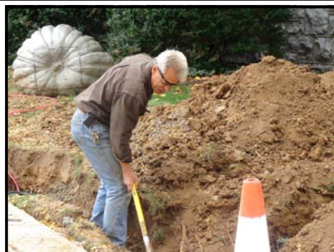
Landscape Worker, Bernie Halterman, installing irrigation at Duke Hall
