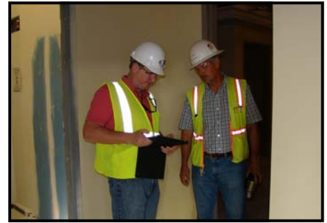
Capital Outlay Project Engineer, Rick Miller at the North Campus construction site
