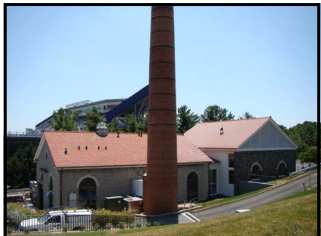
Power Plant renovation
