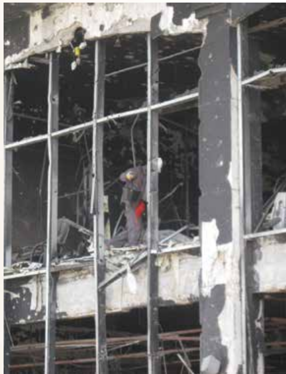
A DCA searcher checks severe damage to a building. The building includes a great deal of blast damage and collapse in some areas. An item of UXO was found on the roof of this building.
