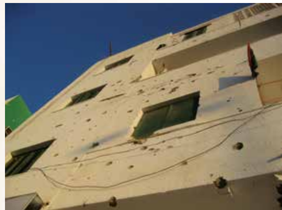
An example of low amounts of battle damage. No items of UXO were found around this building.
