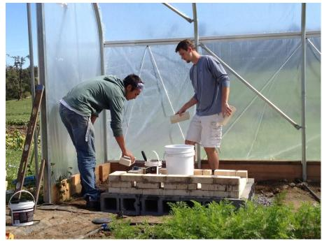
improved through design change in the door to reduce smoke loss from the biochar chamber and increase heat capture by the thermal mass of the unit. Biochar is the product of pyrolyzing biomass, or heating the biomass in an oxygen deprived environment. The biochar was used as a soil amendment in tests as well as stream remediation studies to analyze the potential benefits.
