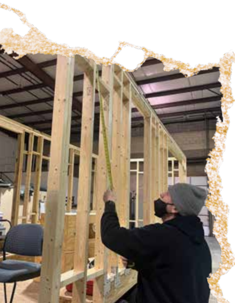
Trevor Ferares measures the trailer walls.
