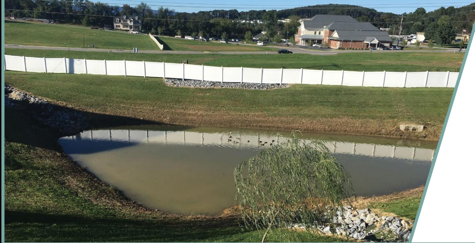
The wet pond/basin located in the Aspen Heights development in Harrisonburg, VA which was mapped using GPS coordinates and eventually transferred to a shape file that is included in the Stormwater GIS layer for tracking and maintenance.
