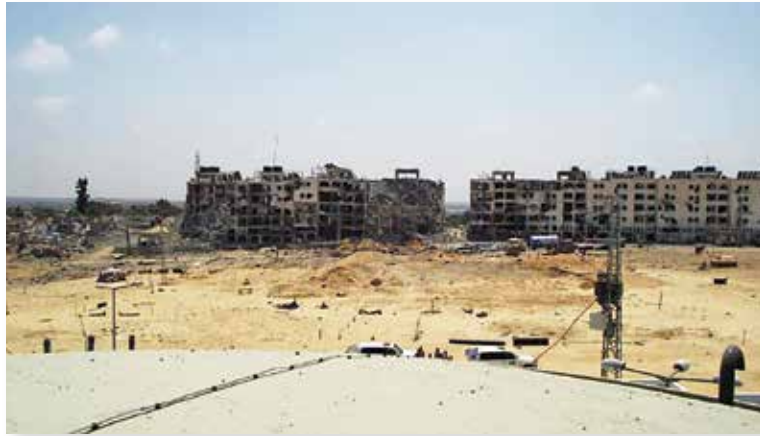
Extent of ERW damage in the residential area in Beit Lahiya, Gaza. All graphics courtesy of UNMAS.
