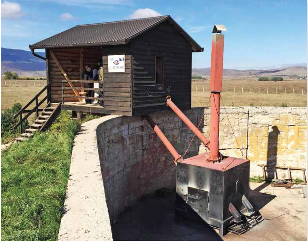
Personnel load items into the furnace via one of two chutes. Gas burners below furnace raise internal temperature above 250 degrees Celsius (482 degrees Fahrenheit).
