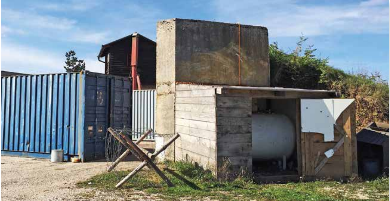
Earth, concrete and steel containers form a concave barrier away from personnel in the chute structure.
